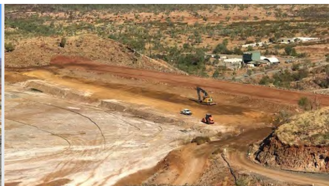
Image 5: Construction of the Savannah Tailings Storage Facility 3m wall lift completed in November 2018
