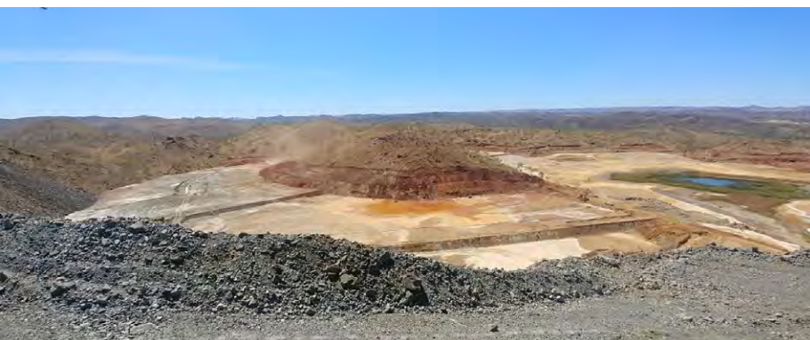
Image 5: Construction of the Savannah Tailings Storage Facility 3m wall lift completed in November 2018
