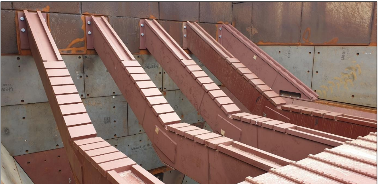
Photo 1 - Refurbished ROM ore bin
