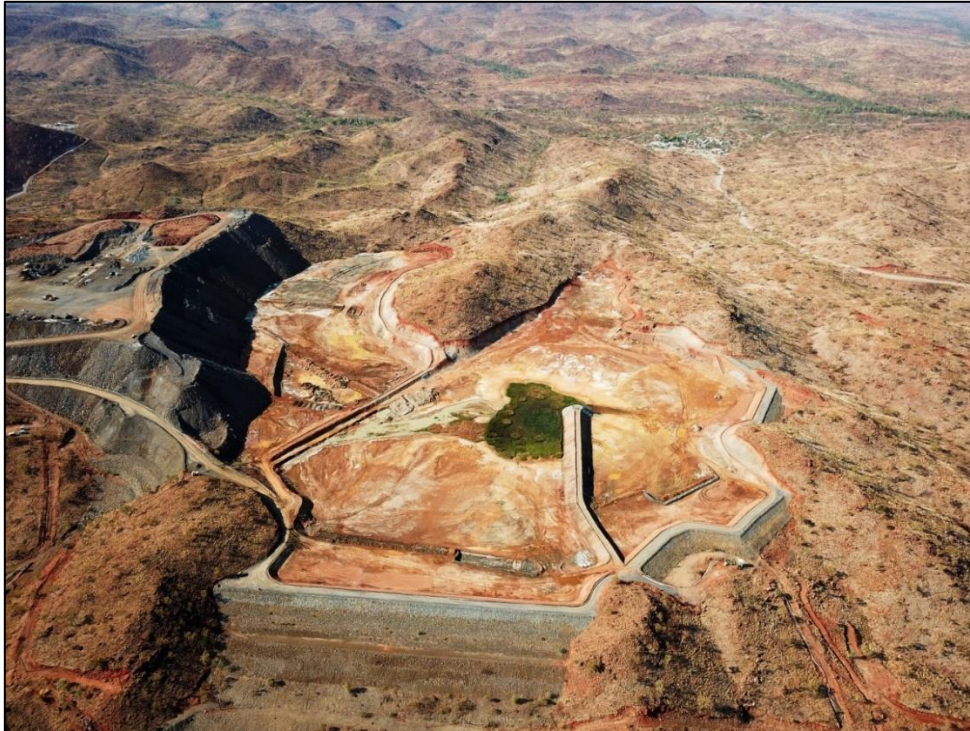
Photo 6 – New 3m wall lift on the tailings storage facility
