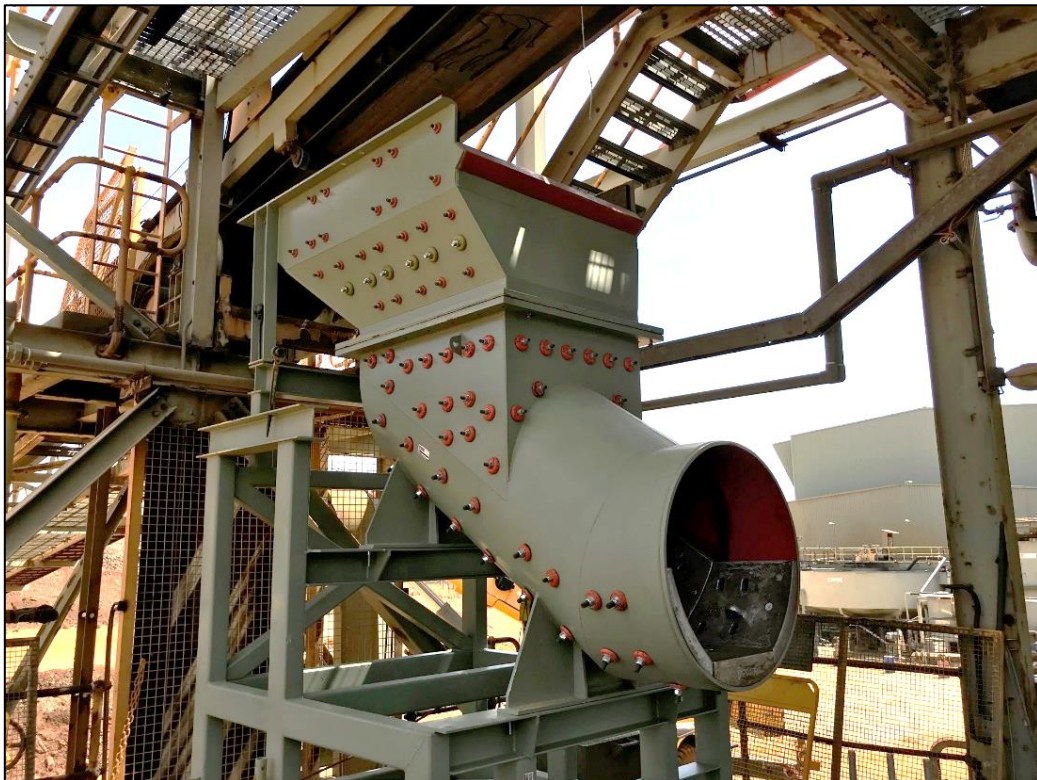
Photo 3 - New SAG mill feed chute
