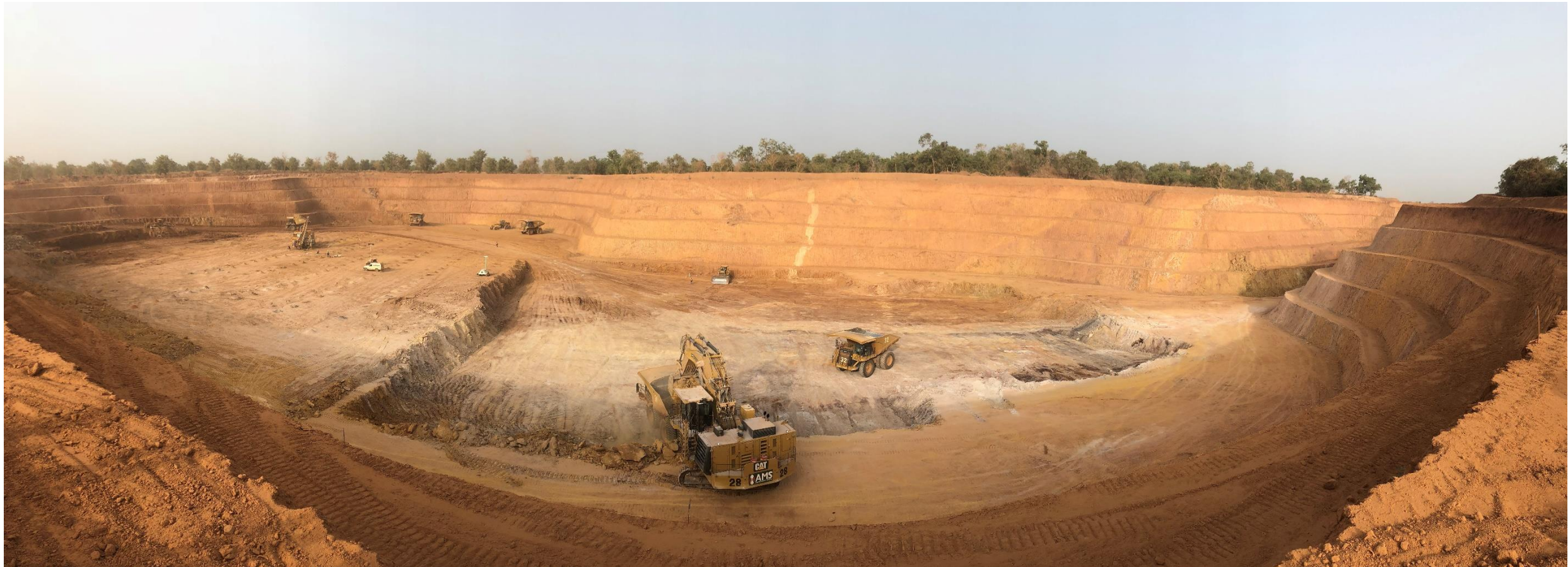
Namakan Pit at Tabakoroni – March 2019
