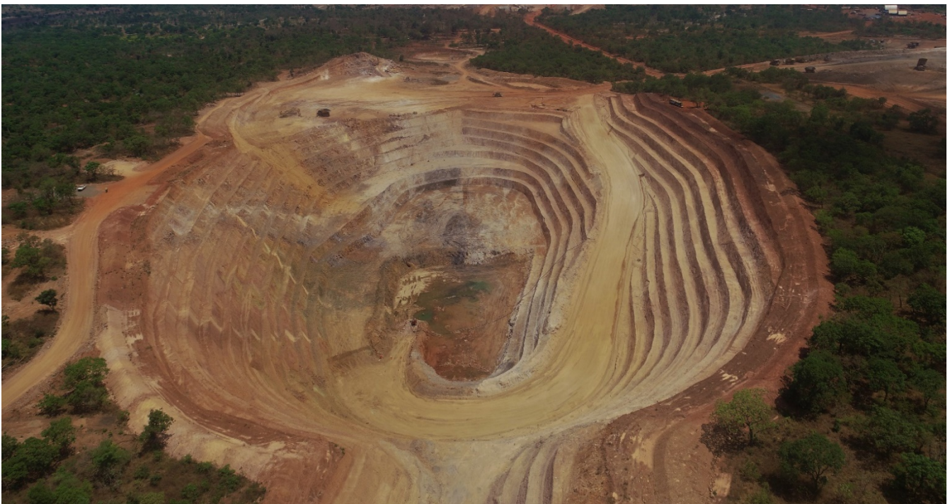
Figure 3: Stage 1 of Namakan Pit at Tabakoroni (north view); stripping of Stage 2 of the pit is underway (top of image)
