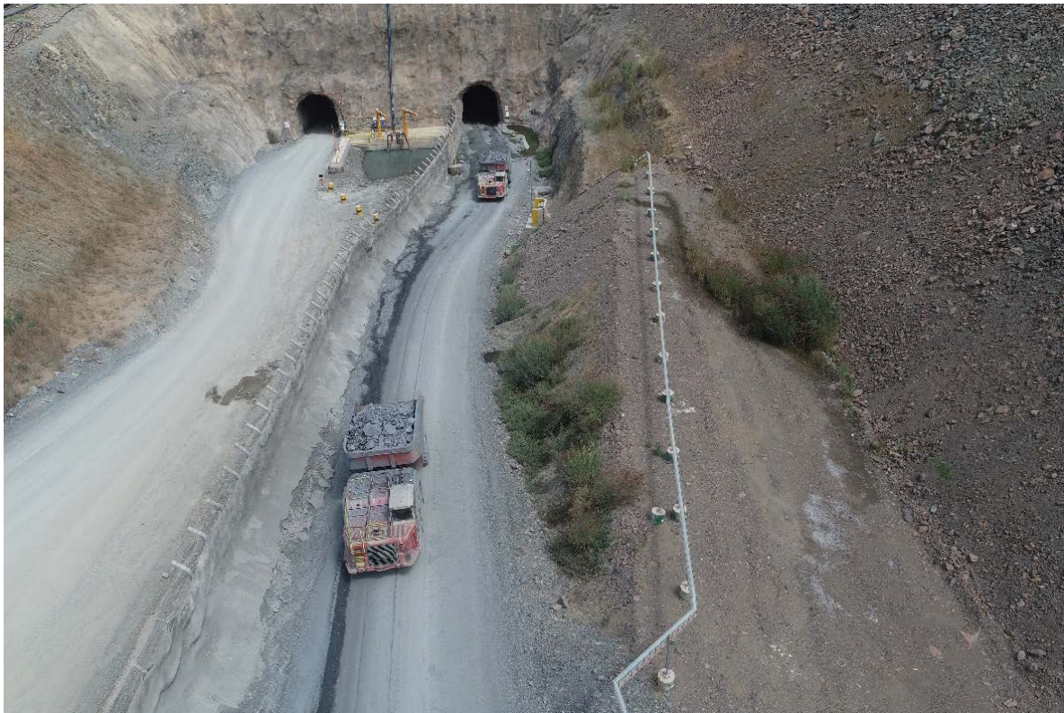
Figure 4: Automated Haul Trucks leaving the Syama Portal
