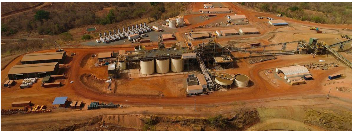
Figure 6: Mako Processing Plant
