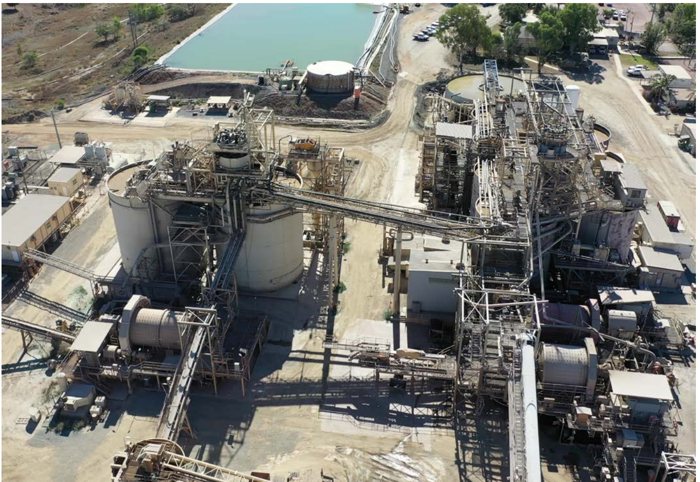
Figure 1: Nolans Processing Plant with third grinding mill (Mill #3) to be recommissioned to the left of picture. Existing grinding mills located in bottom right of picture
