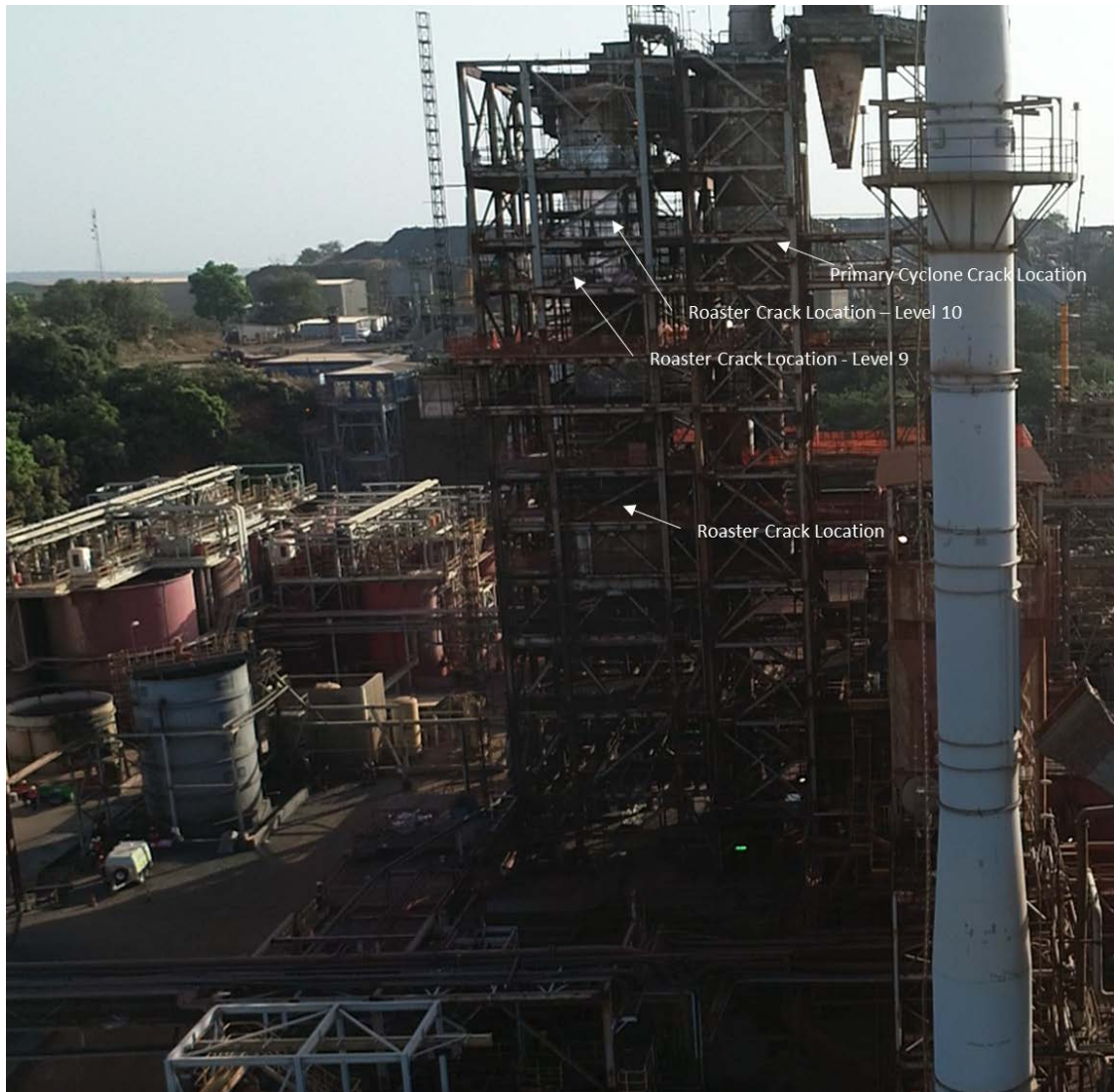
Figure 1: Syama Roaster showing repair locations
