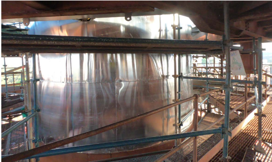
Figure 3: Syama Roaster repair completion
