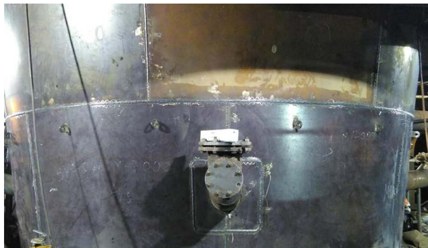
Figure 2: Syama Roaster steel replating
