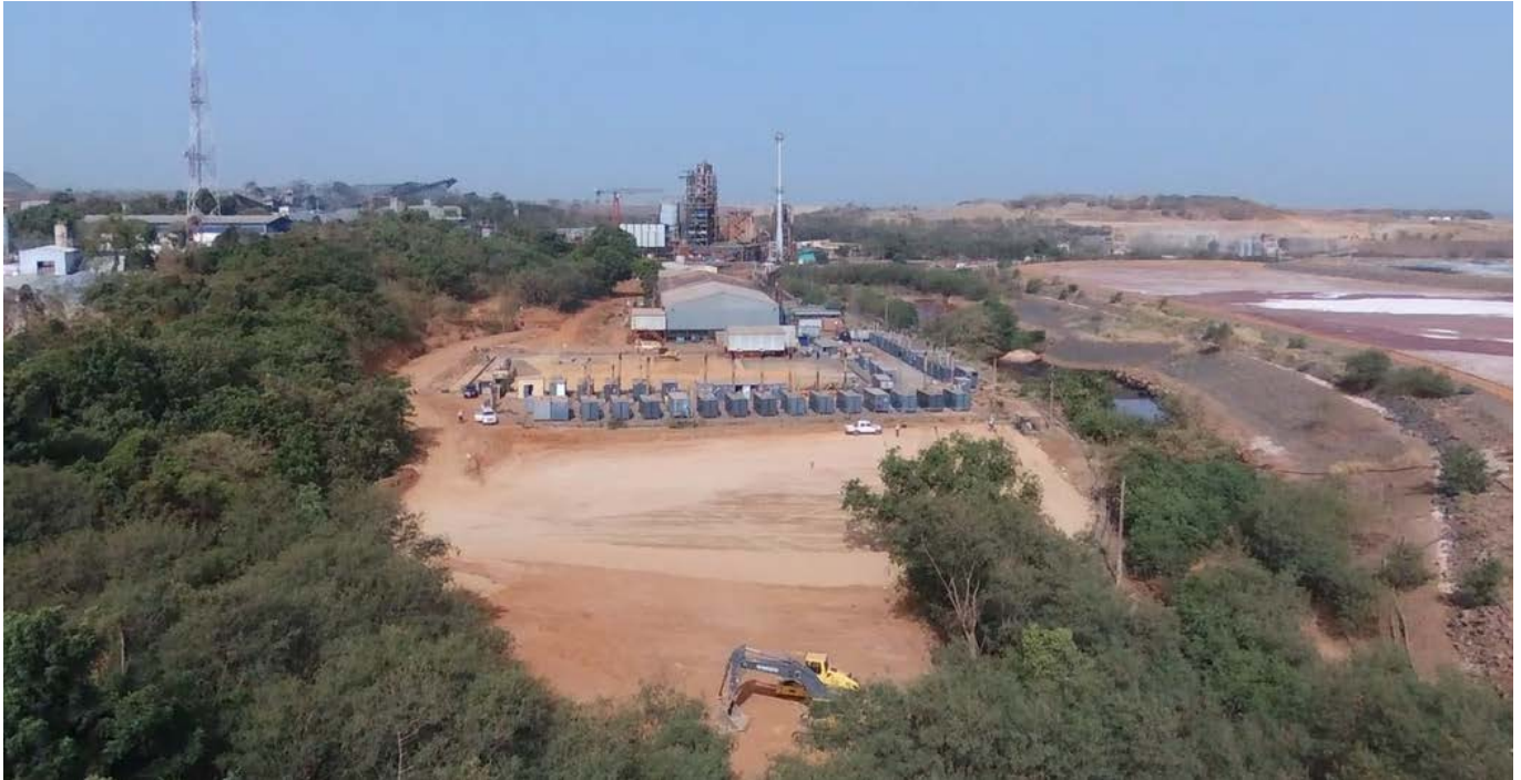
Figure 5: Earthworks commenced at the new Syama Solar-Hybrid Power Station
