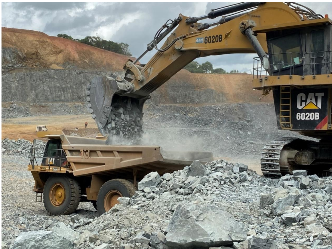
Figure 3: Recently commissioned Caterpillar 6020B excavator in operation at Mako
