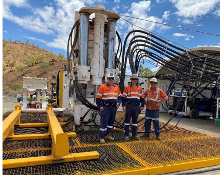
Figure 1: RUC Raisebore rig setting up on the surface
