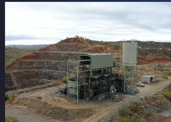
Paste plant operational
