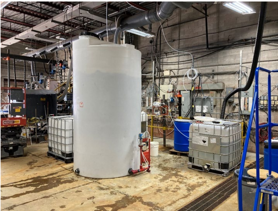
Figure 5: Bulk 5T column of ore being leached, with PLS collected in IBC's ready for the neutralisation and refining stage.
